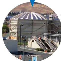
Delta Diablo would receive trucks of feedstock from MDRR, and anaerobic digesters would co-digest it with municipal wastewater sludge to create renewable biogas and biosolids.
